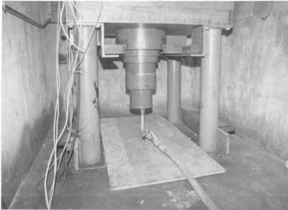
Figure 5.18. Primary grouting from lower anchorage
