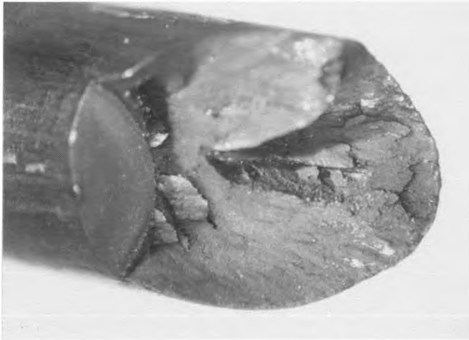
Figure 5.34 Outer wire failure in stay lengths, strand 18
