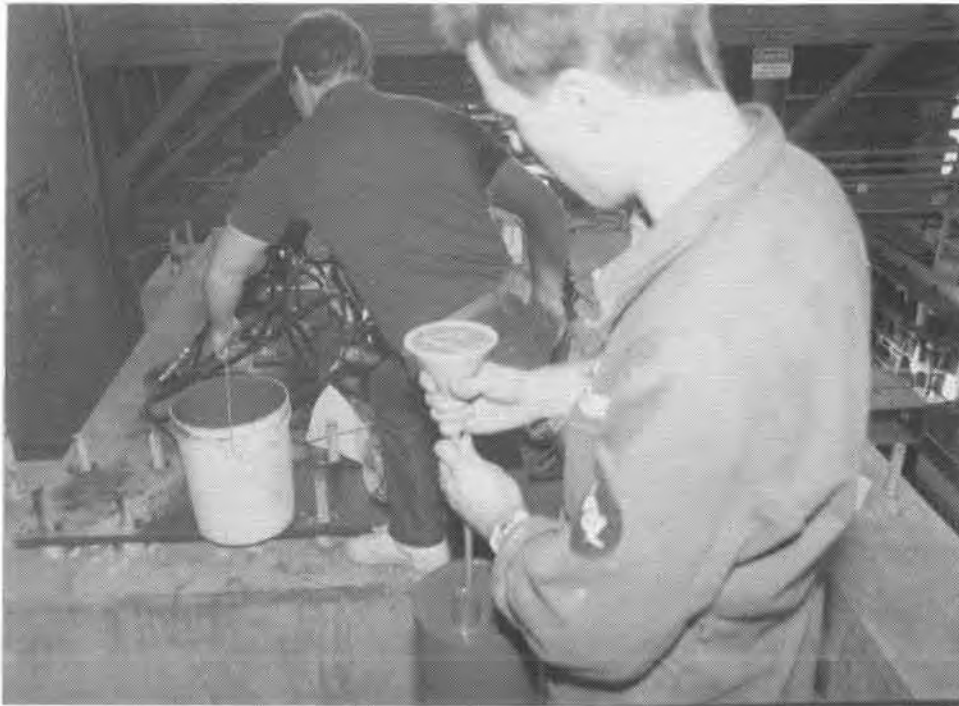
Figure 5.20. Secondary grouting procedure
