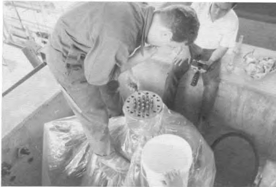
Figure 5.19. Siphoning of bleed water from top anchorage
